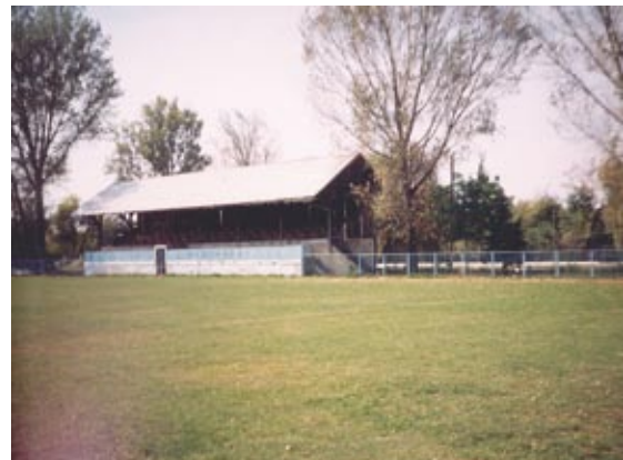
Site 1 – Building III
